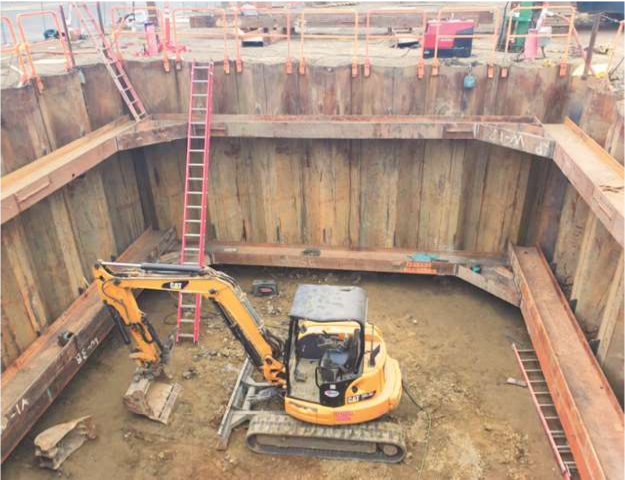
ETSU Phase 1A - New Pump Station
