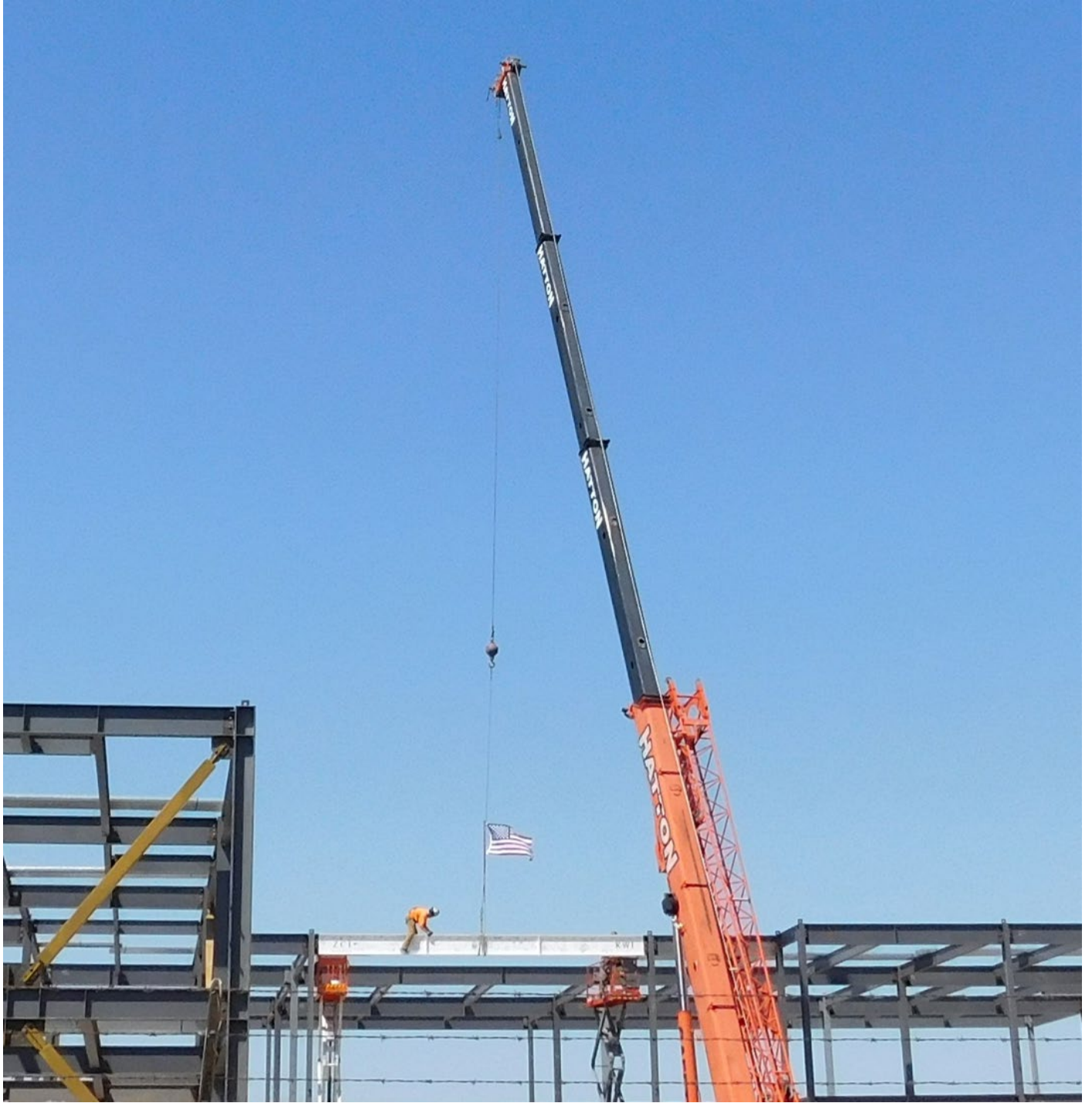
Placement of the Topping Beam on the New Campus Building Cover Picture: ETSU Aeration Basin Construction
