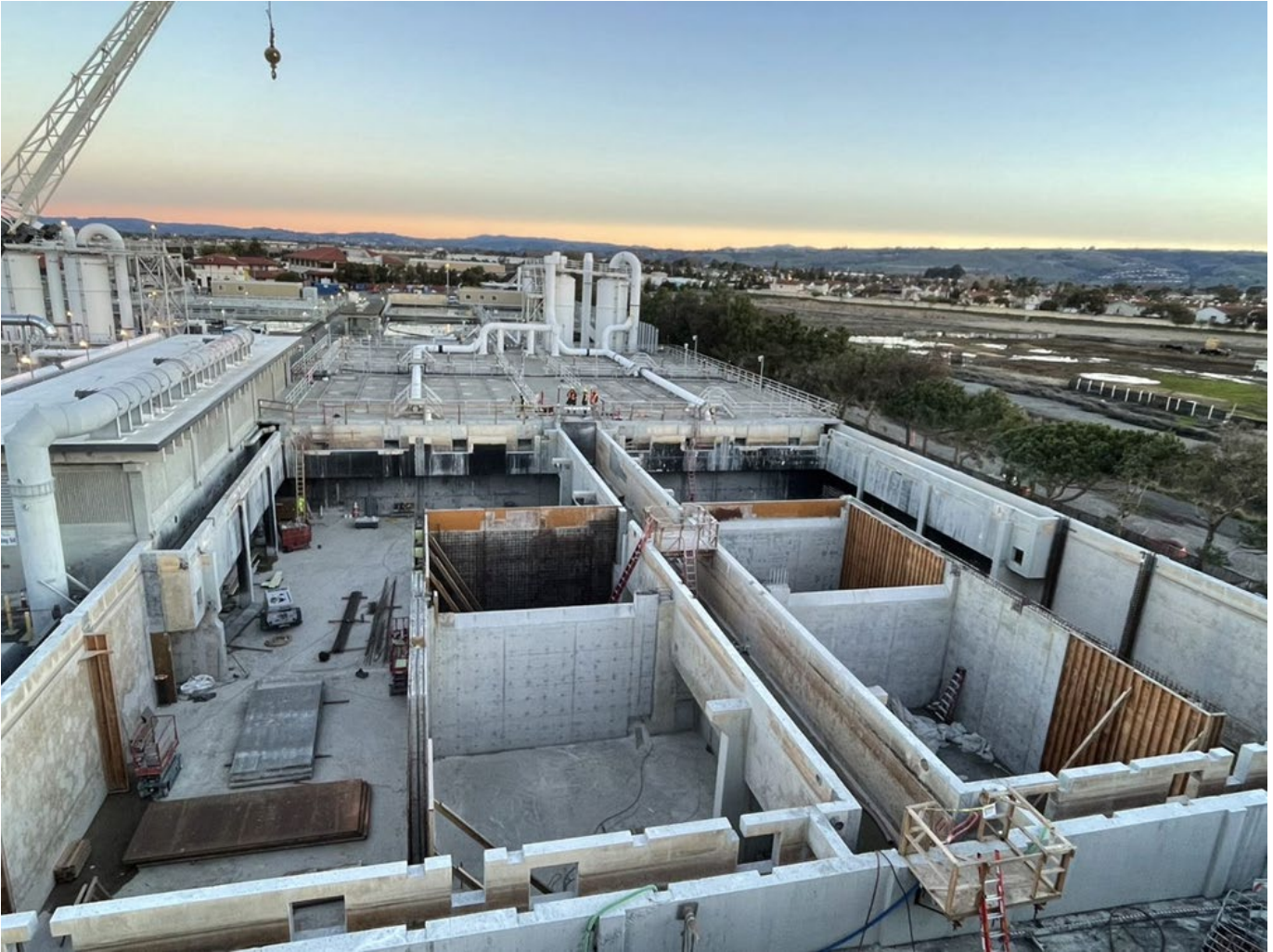
ETSU Aeration Basin Construction
