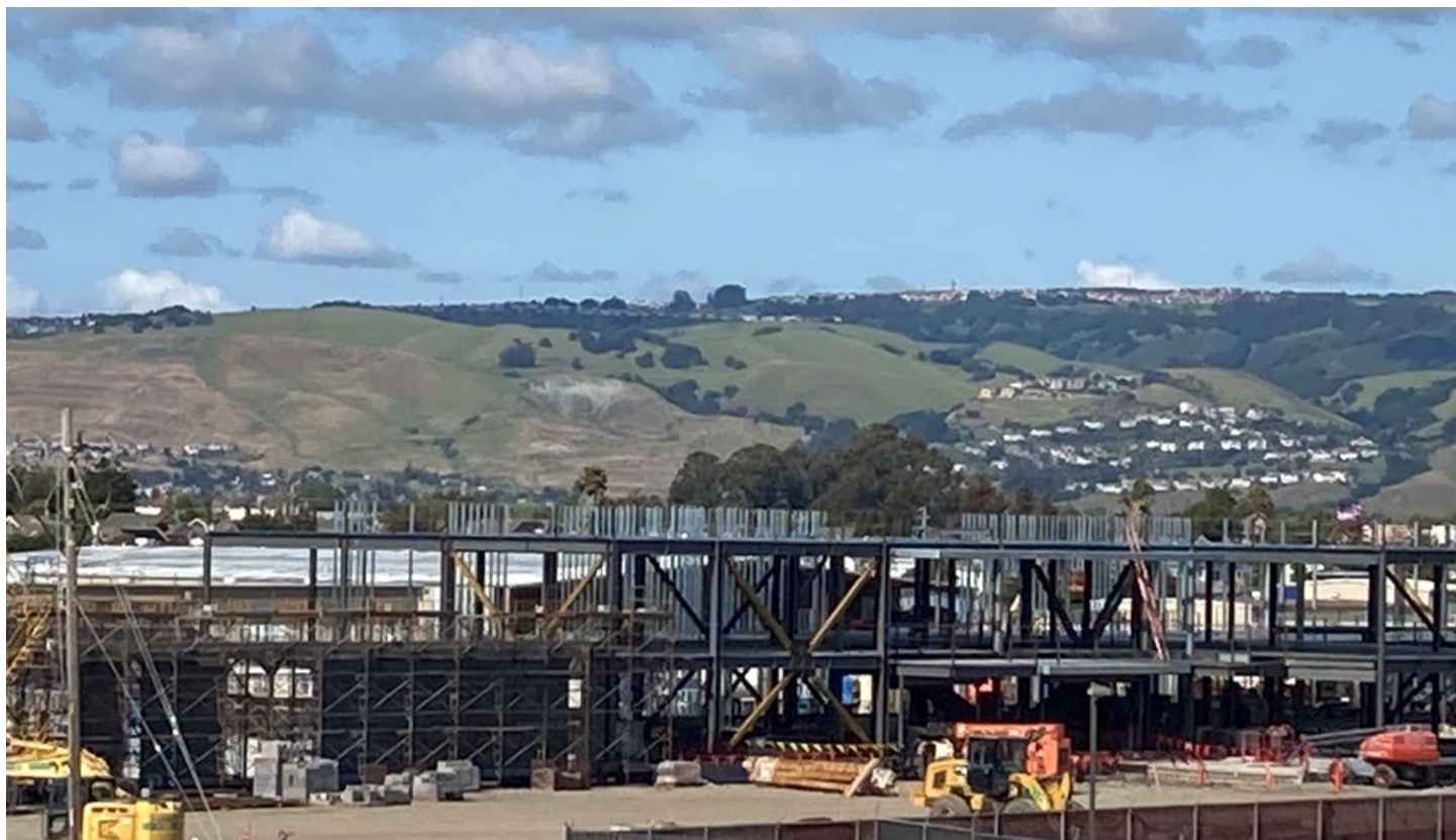
Structural Steel for the New Campus Building
