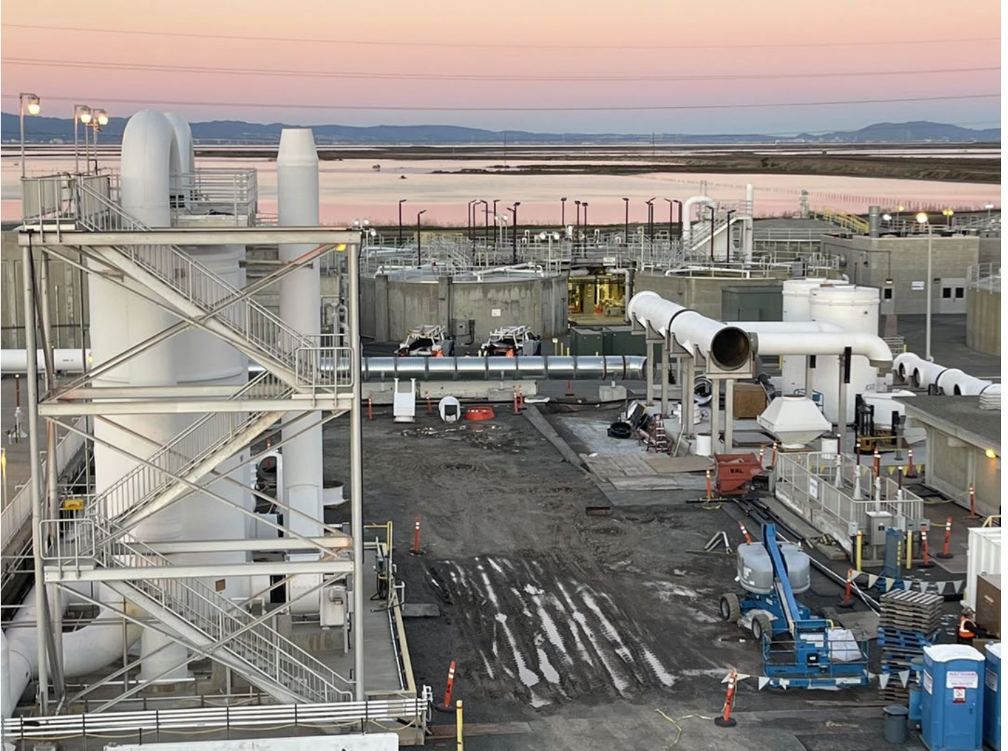
ETSU Aeration Basin Construction
