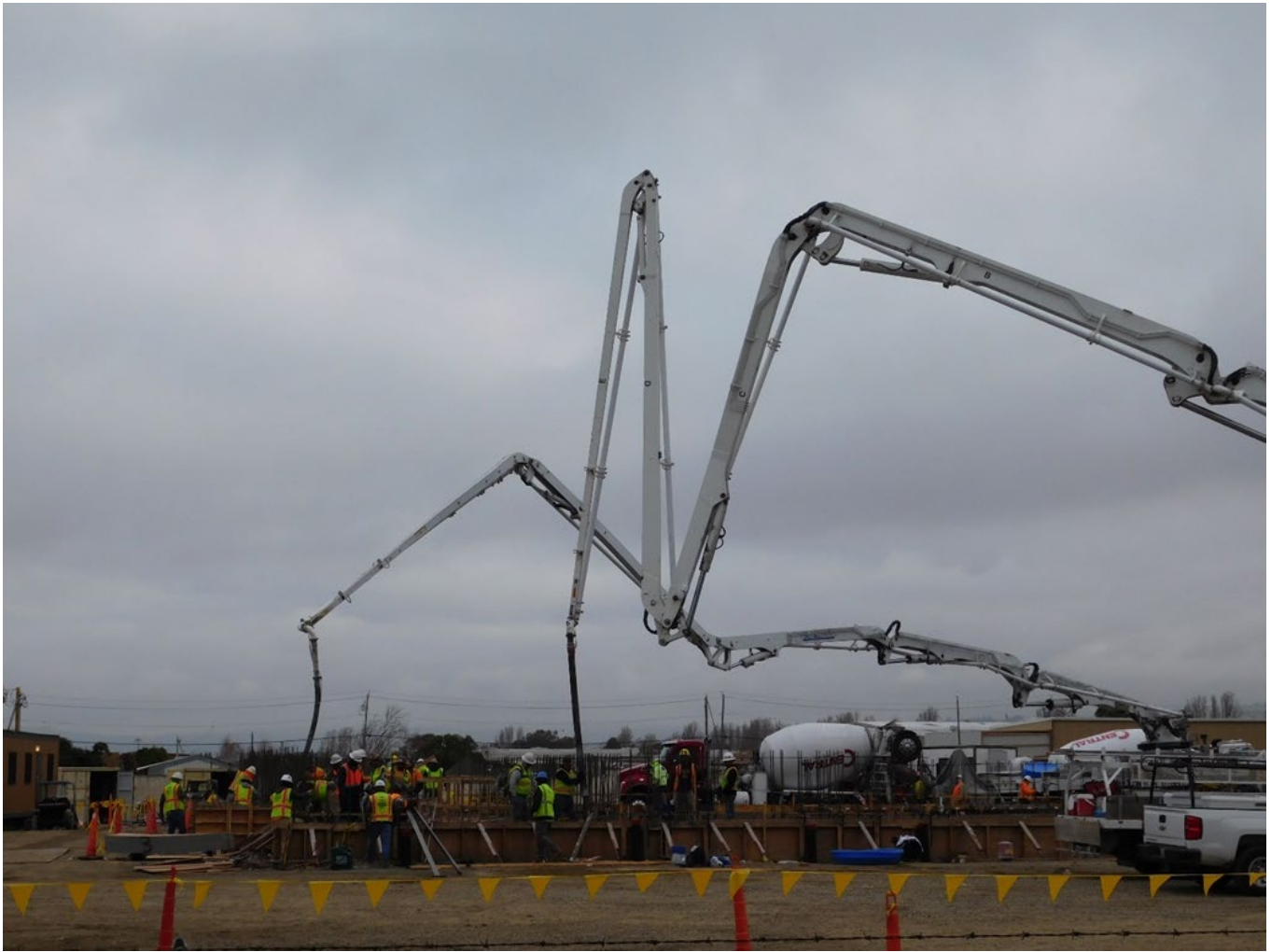
Pouring Concrete for the New Campus Building
