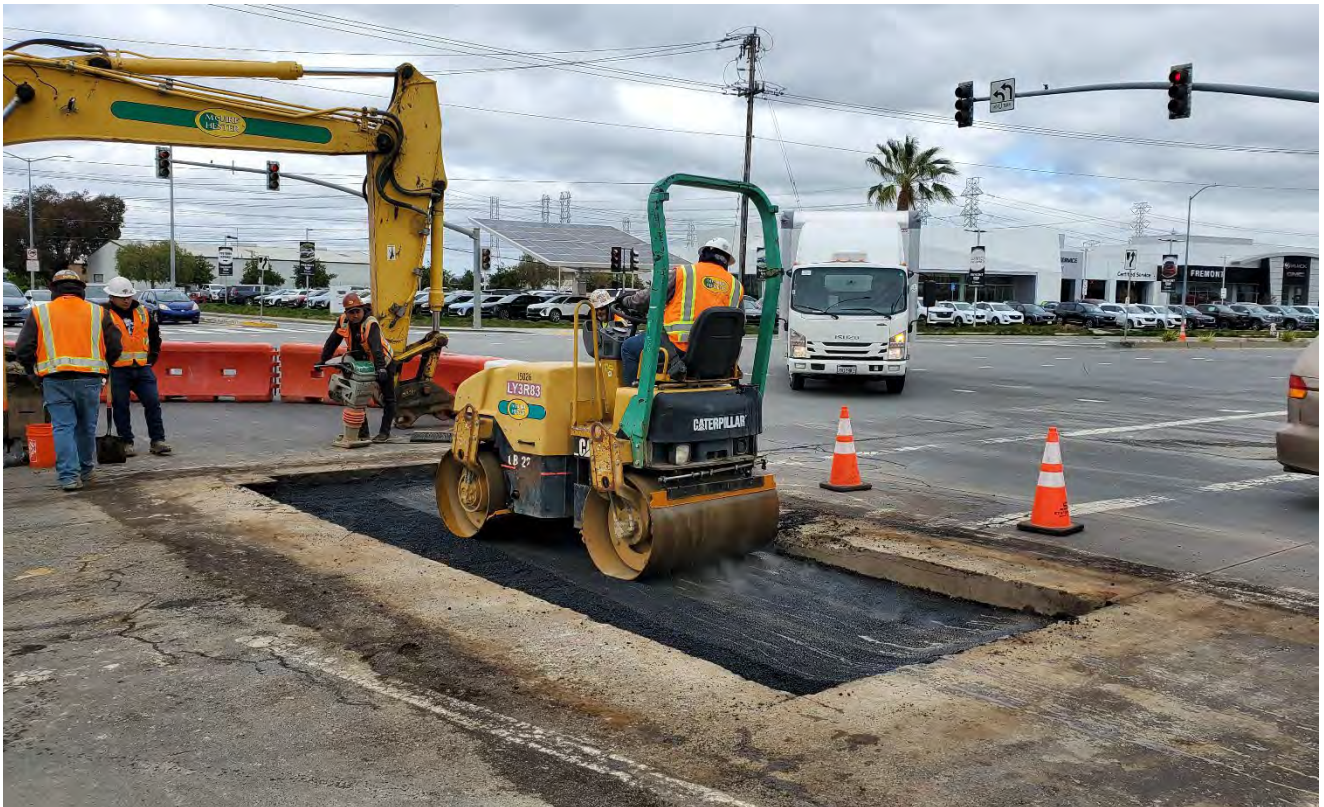
Figure 6 – Placement of Asphalt for Westernmost Section
