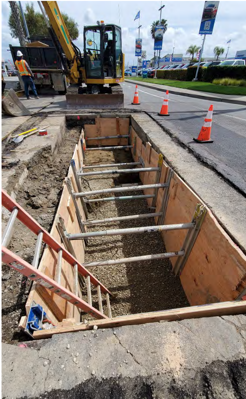
Figure 8 – Excavation of Easternmost Section
