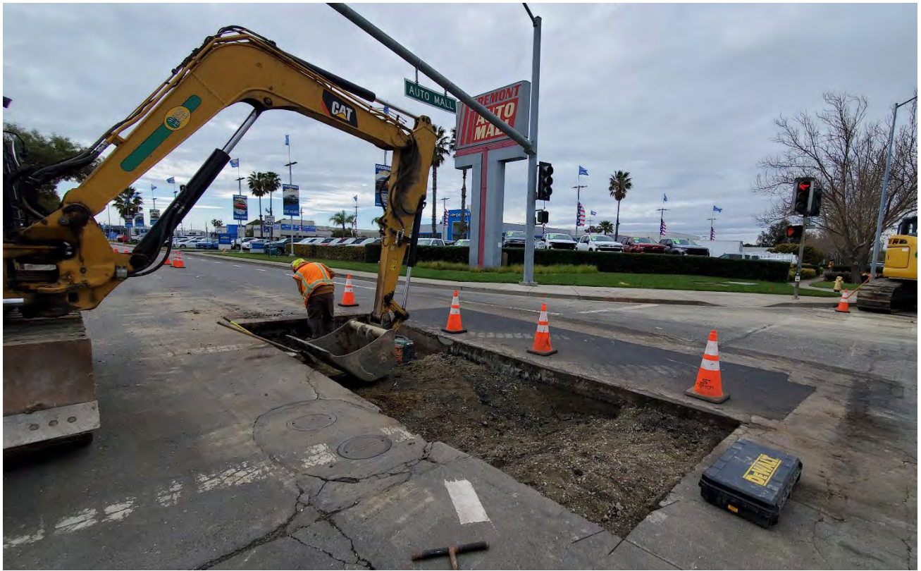
Figure 7 – Excavation of Easternmost Section
