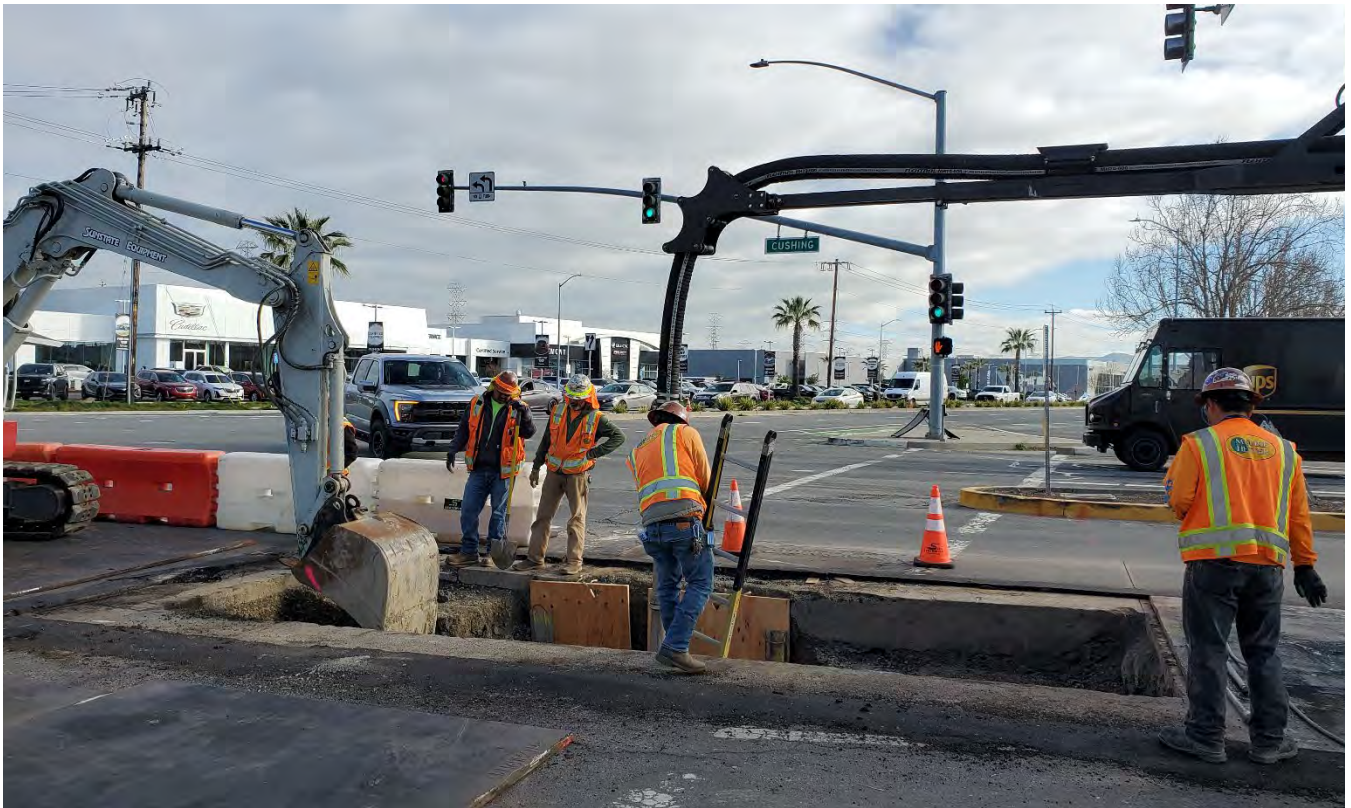
Figure 3 – Excavation of Westernmost Section
