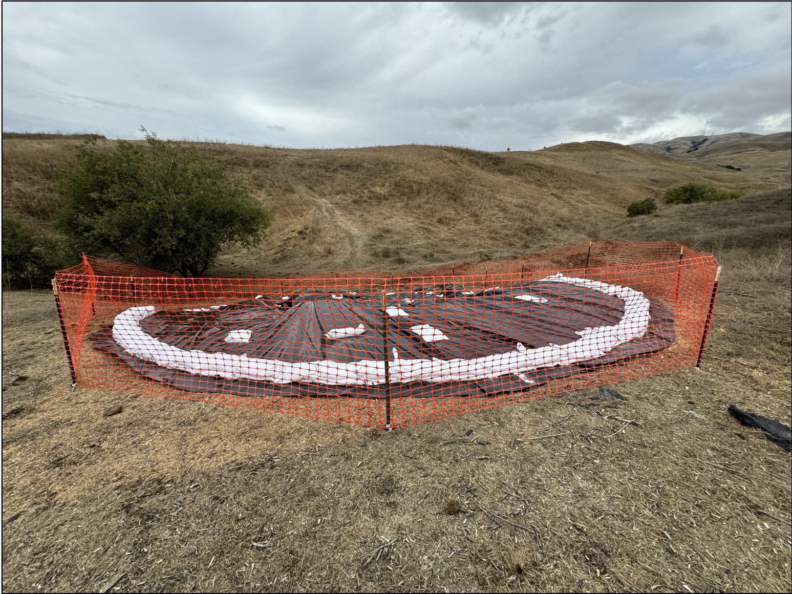
Figure 6 - Manhole G24006 - Temporary Slope Protection - Looking North
