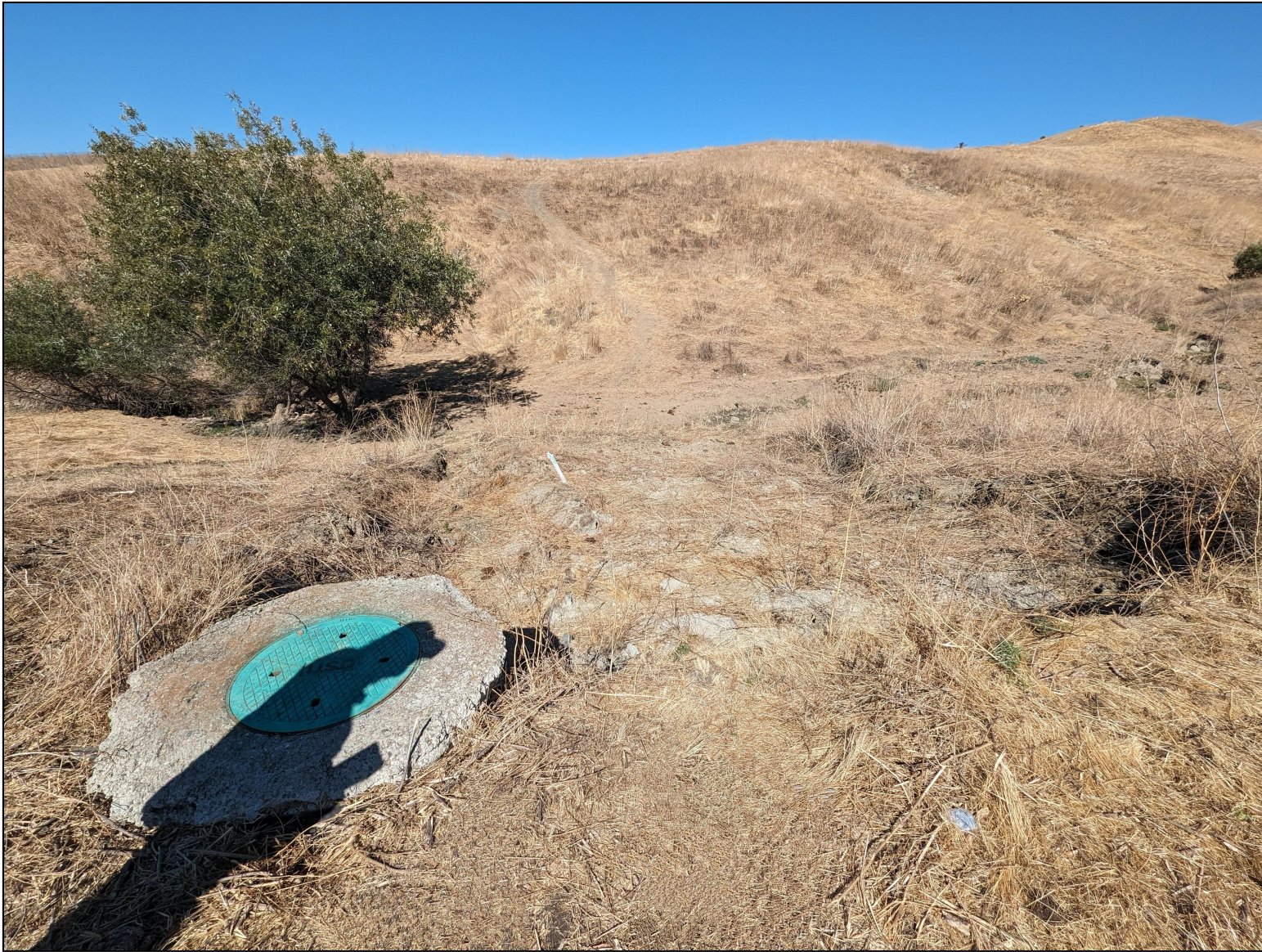
Figure 4 - Manhole G24006 - Before Installation of Slope Protection - Looking North
