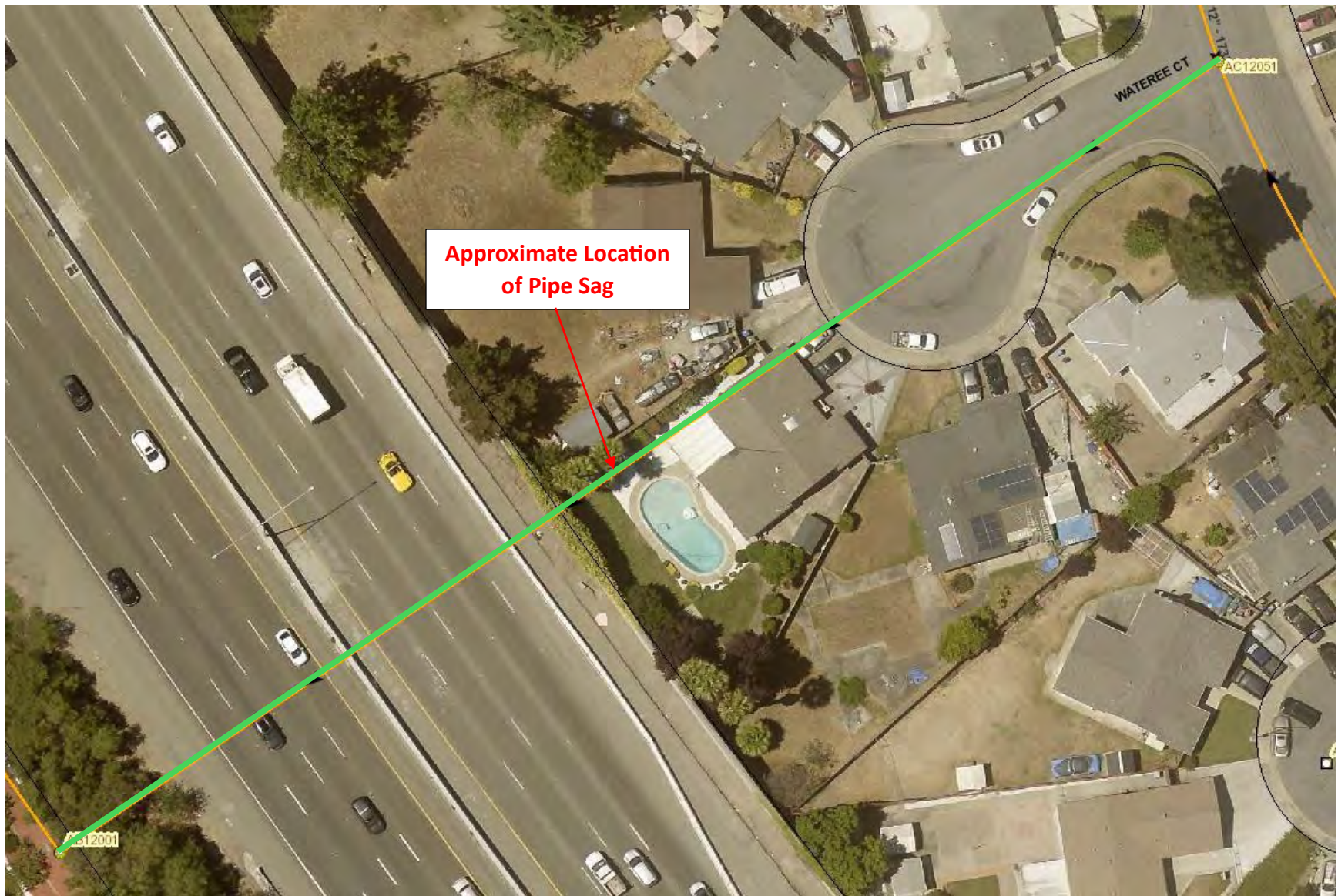
Figure 3 – Site No. 6 (Waterree Court) – Moderate to Severe Sagging
