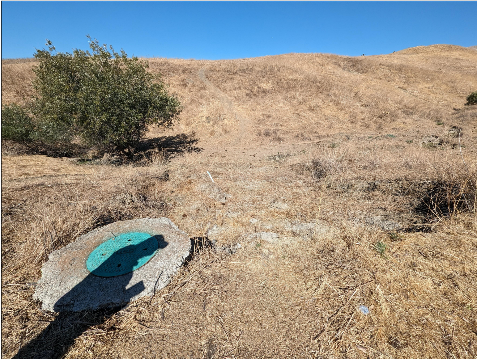
Figure 5 - Manhole G24006 - Before Installation of Slope Protection - Looking North
