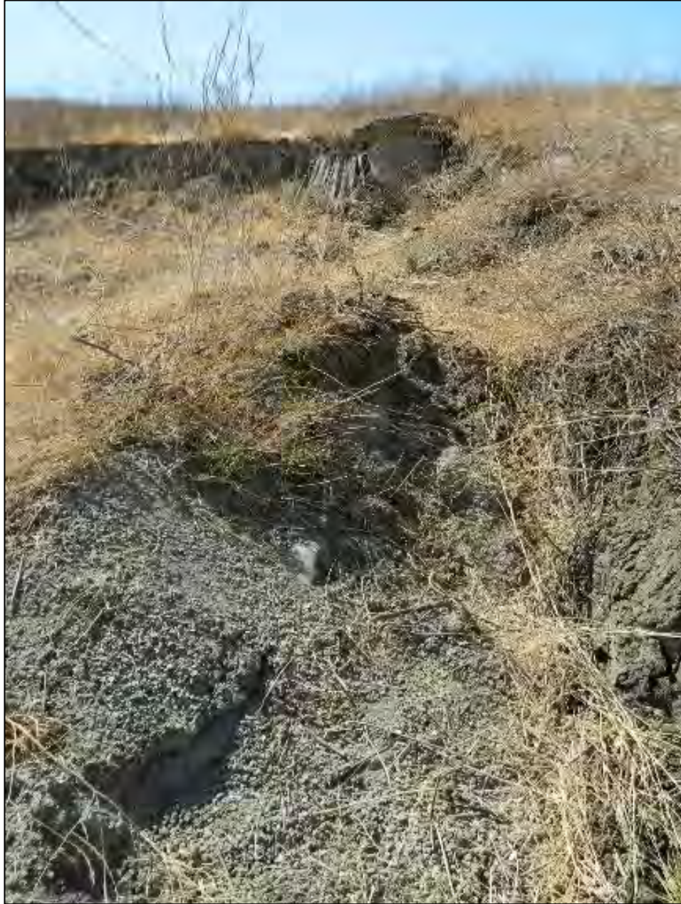
Figure 6 - Manhole G24006 - Before Installation of Slope Protection - Looking South
