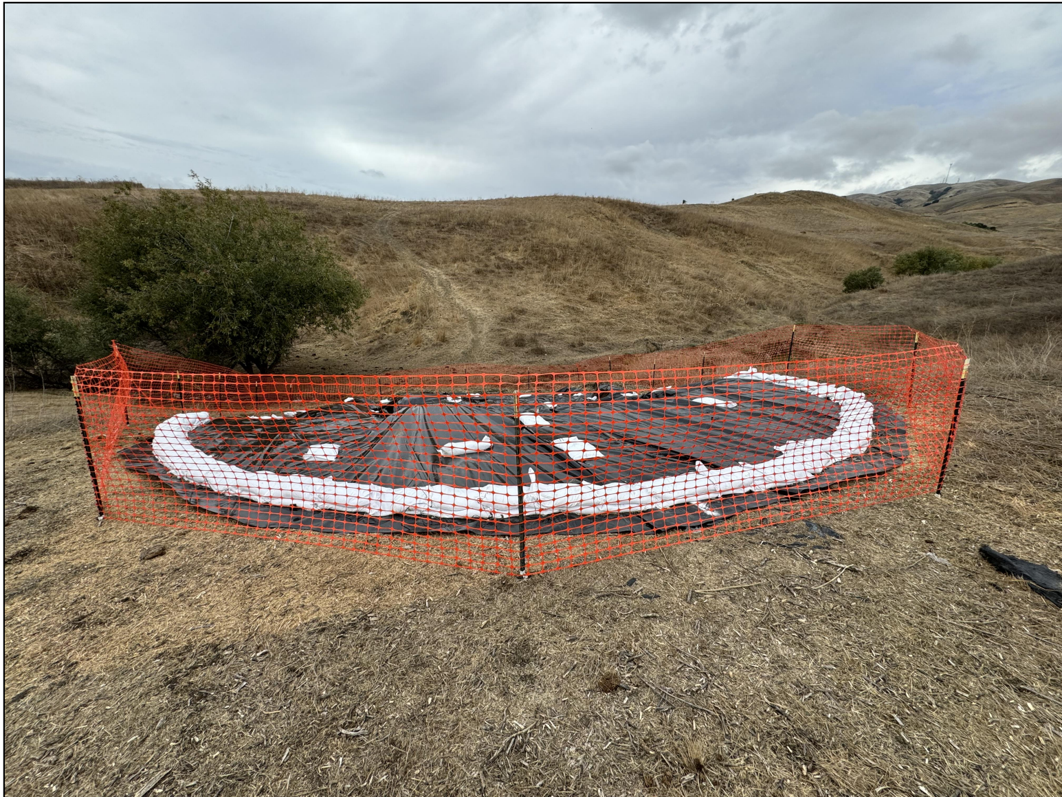
Figure 7 - Manhole G24006 - Temporary Slope Protection - Looking North
