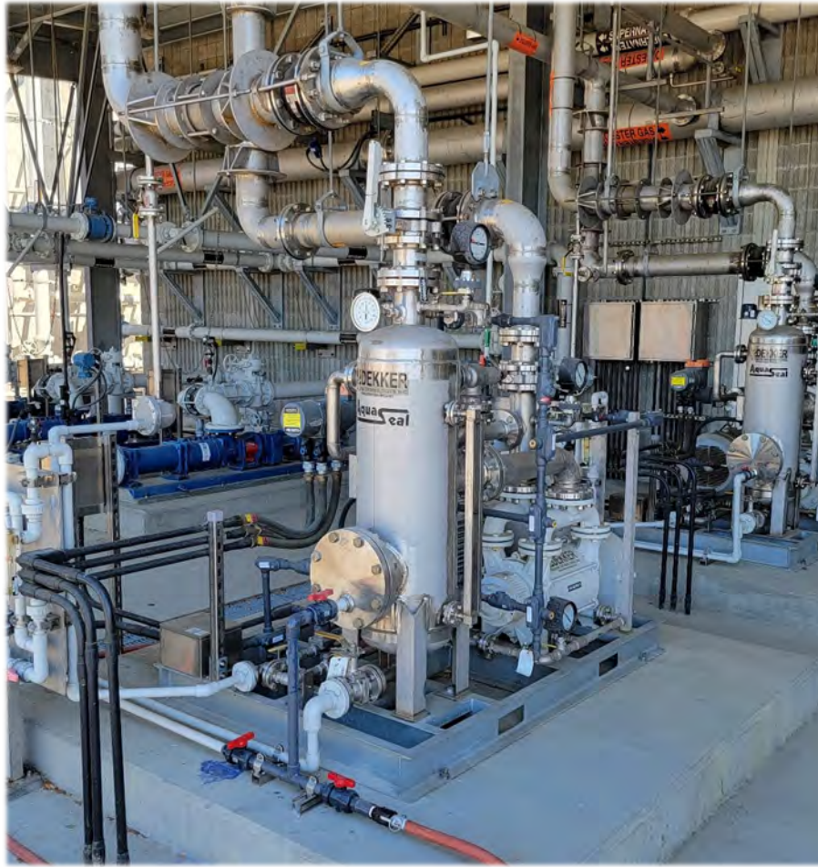
Figure 4 – Gas Lance Mixing Compressors
