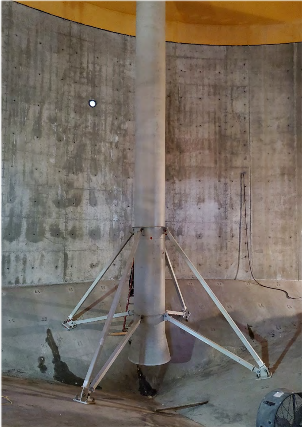
Figure 6 – Gas Lance Mixing Draft Tube
