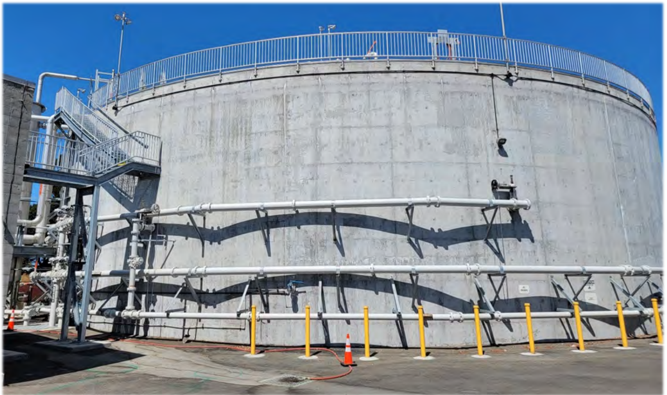
Figure 2 – Primary Digester No. 7 Concrete Tank
