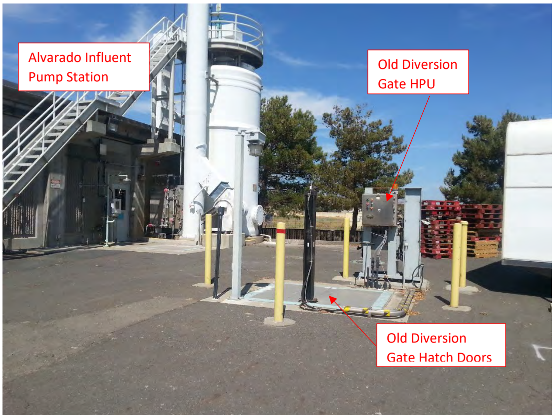
Figure 6 – Old Diversion Gate Box Hatch Doors and Hydraulic Power Unit (HPU)
