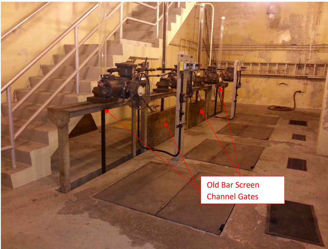
Figure 10 – Old Bar Screen Channel Gates in the Wet Well Room
