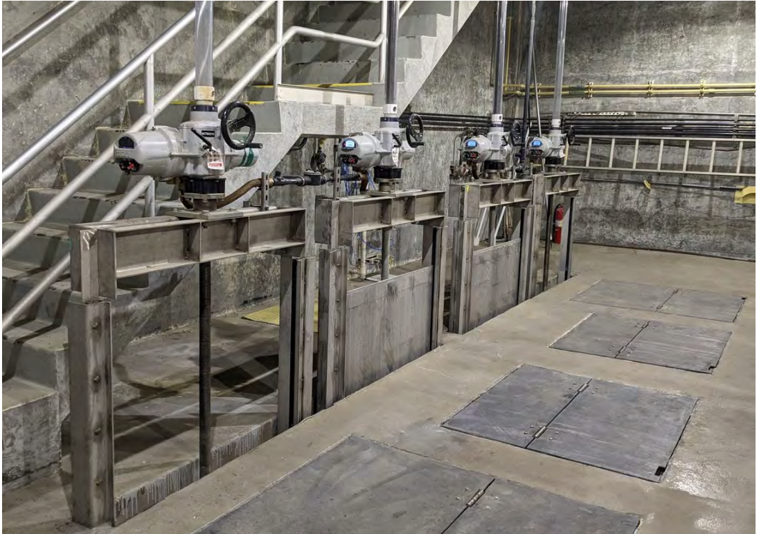
Figure 11 – New Bar Screen Channel Gates in the Wet Well Room
