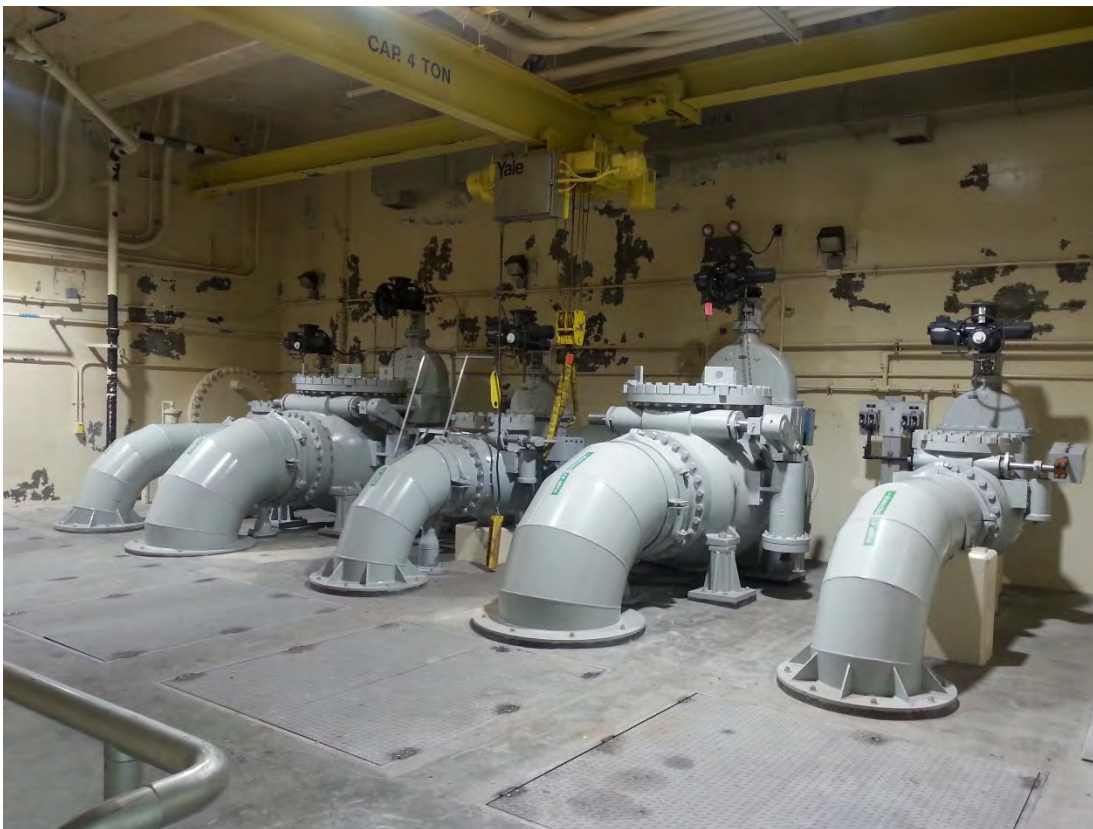
Figure 4 – Old Piping and Valves at the Dry Well Intermediate Level
