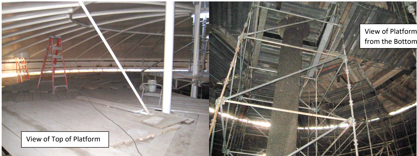
Figure 6 – Scaffolding Platform Inside Primary Digester No. 5
