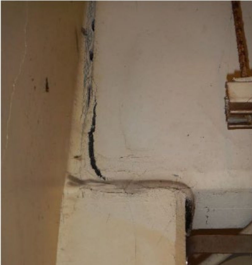
Figure 4 – East Primary Clarifier Building – Multiple Cracked Roof T-beams
