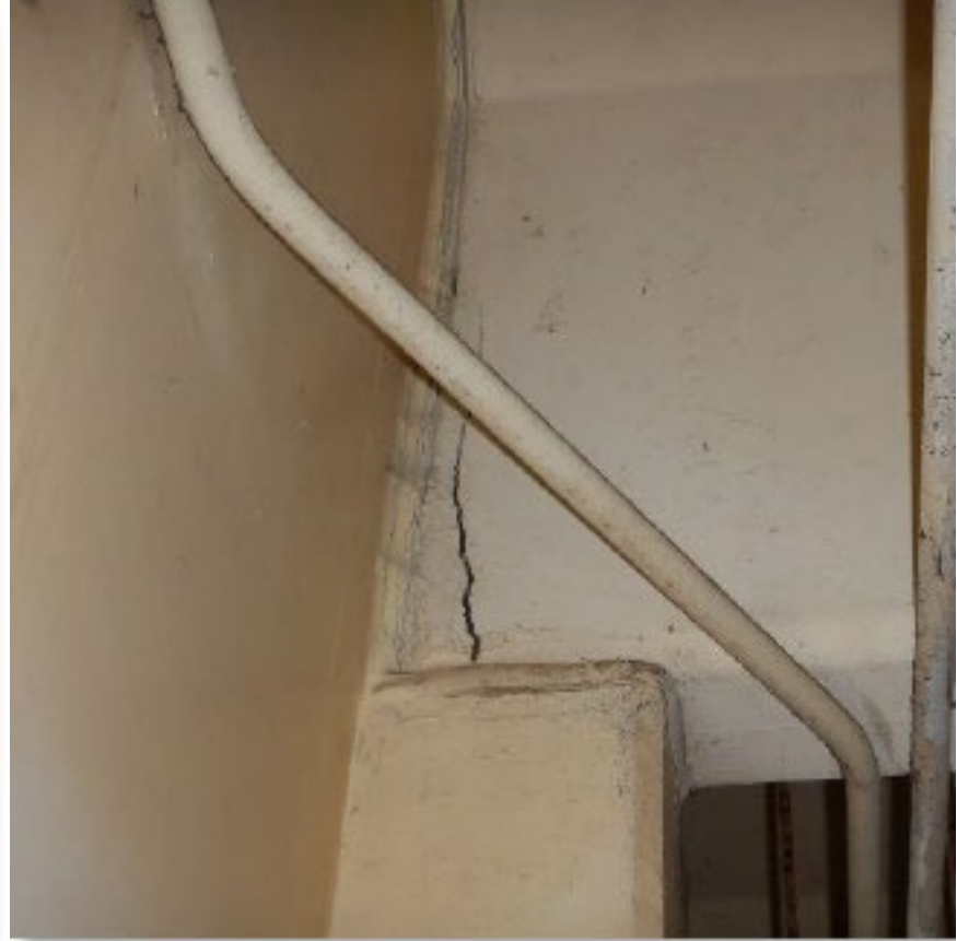
Figure 4 – East Primary Clarifier Building – Multiple Cracked Roof T-beams
