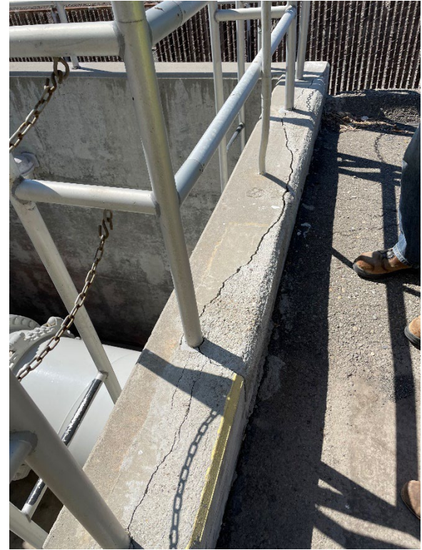
Figure 6 – Alvarado Influent Pump Station Flow Meter Pit – Cracked Curb at Multiple Locations
