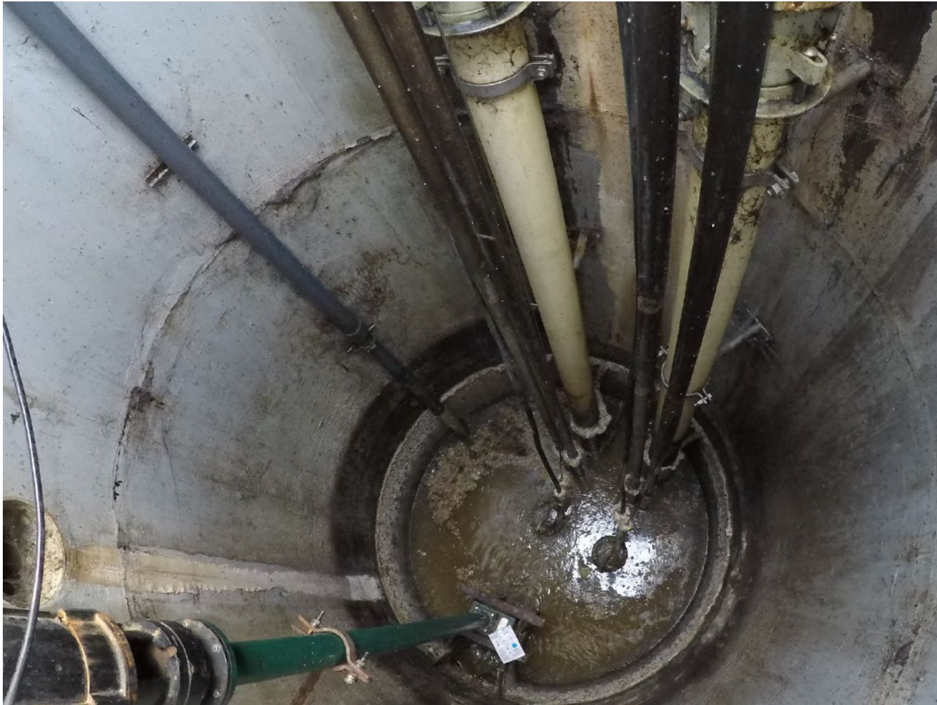
Figure 5 – Existing Wetwell and Pumps
