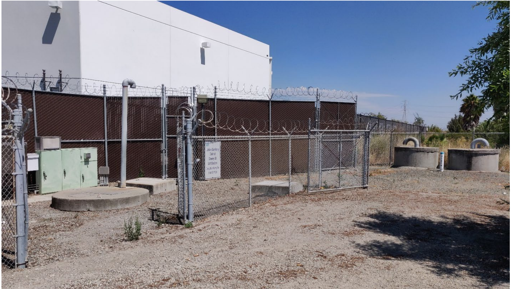
Figure 4 – Cherry Street Pump Station
