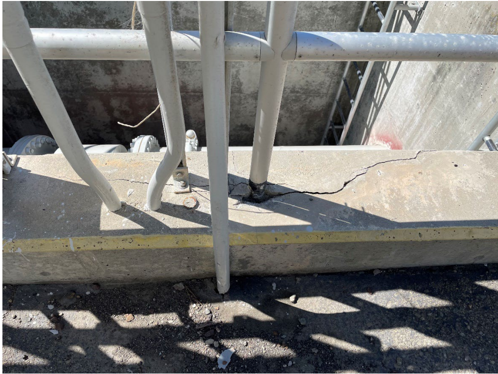
Figure 6 – Alvarado Influent Pump Station Flow Meter Pit – Cracked Curb at Multiple Locations
