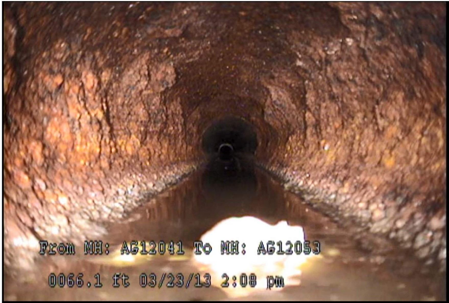
Figure 4 - Site No. 14, Alpine Court, Fremont; Observed corrosion.
