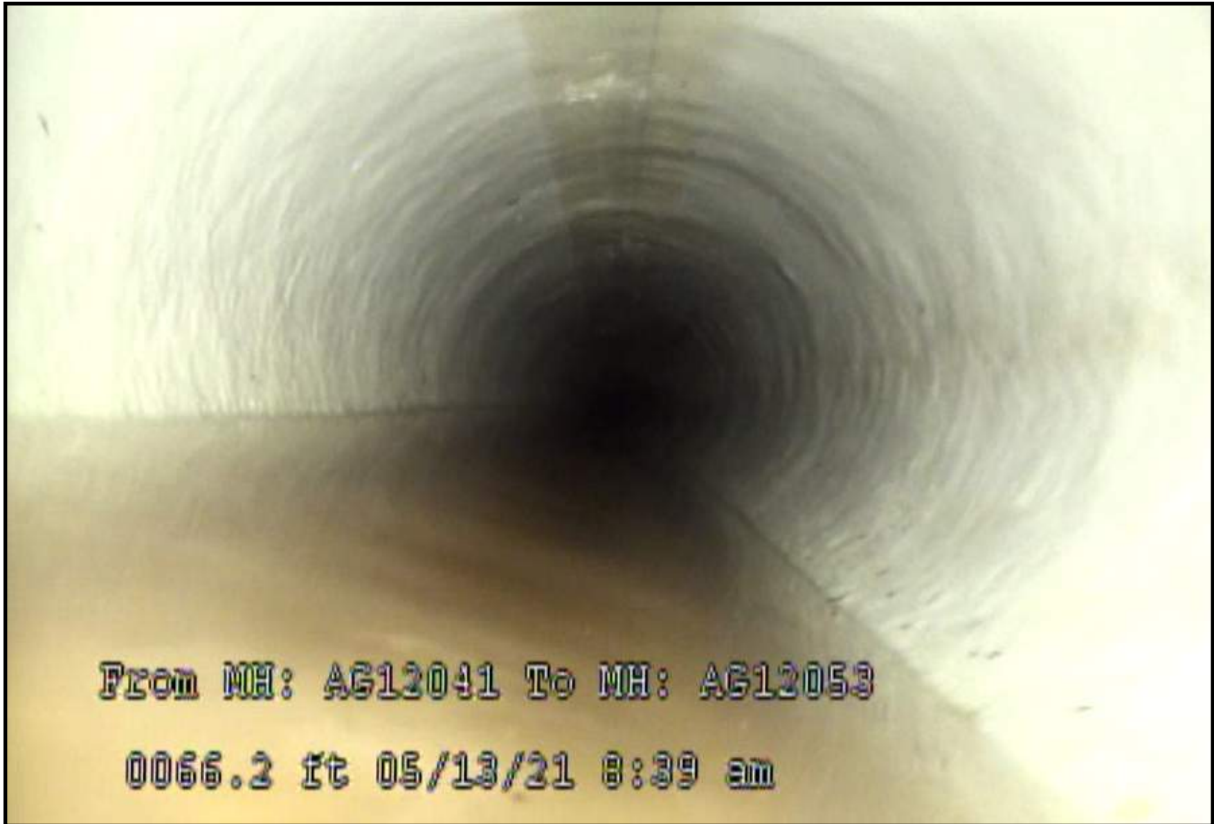
Figure 5 - Site No. 14, Alpine Court, Fremont; CIPP Liner Installed.
