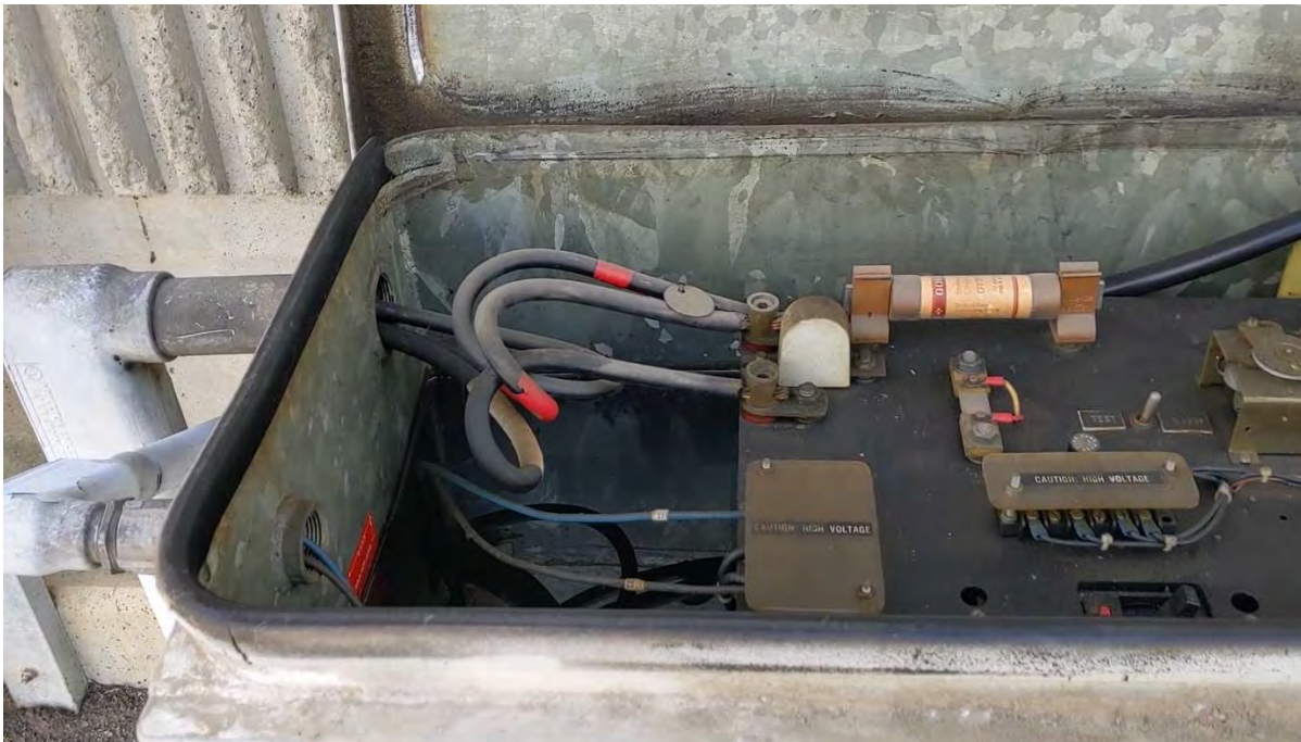
Figure 4 – Interior of Oil-Cooled Rectifier
