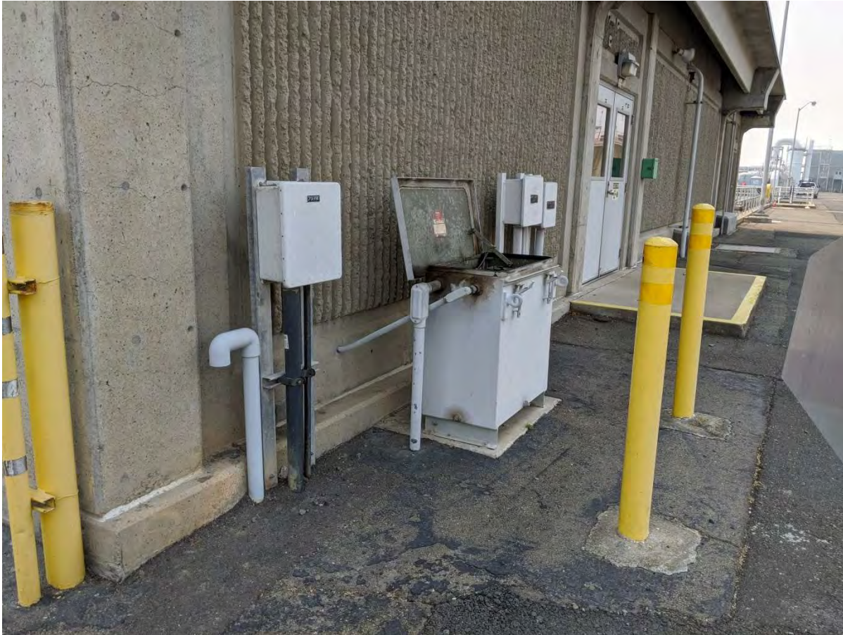
Figure 3 – Existing Oil-Cooled Rectifier at Alvarado Effluent PS
