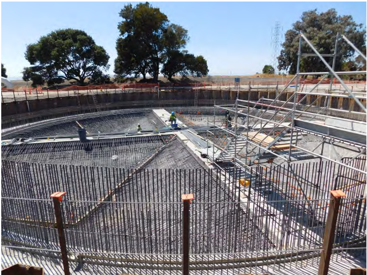
Image: Rebar Installation for Cone-Shaped Base Slabs
