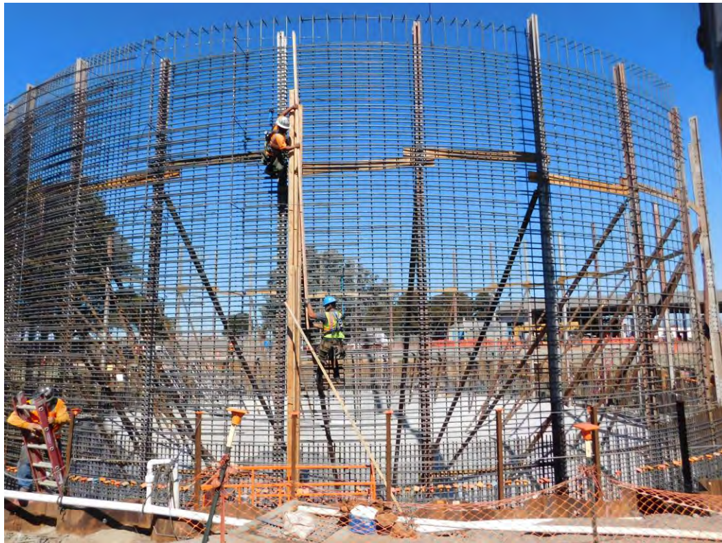
Image: Rebar Installation for Walls
