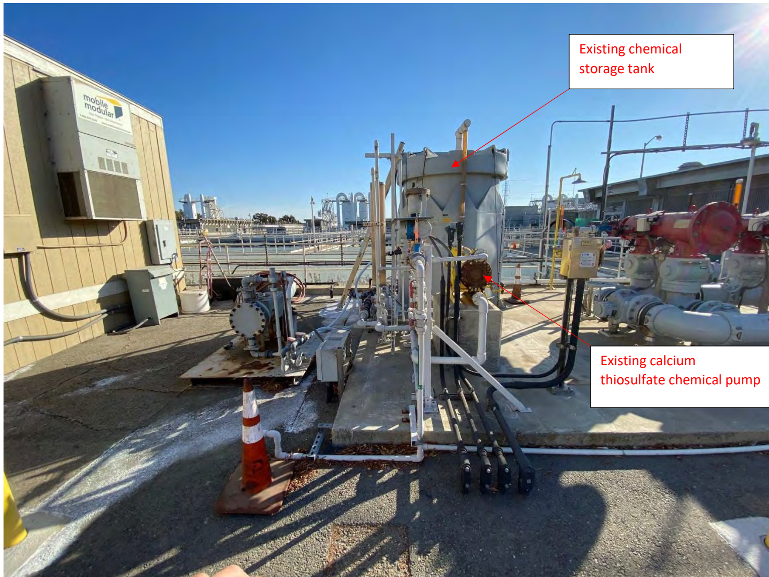
FIGURE 4 – Existing Calcium Thiosulfate Chemical Feed System
