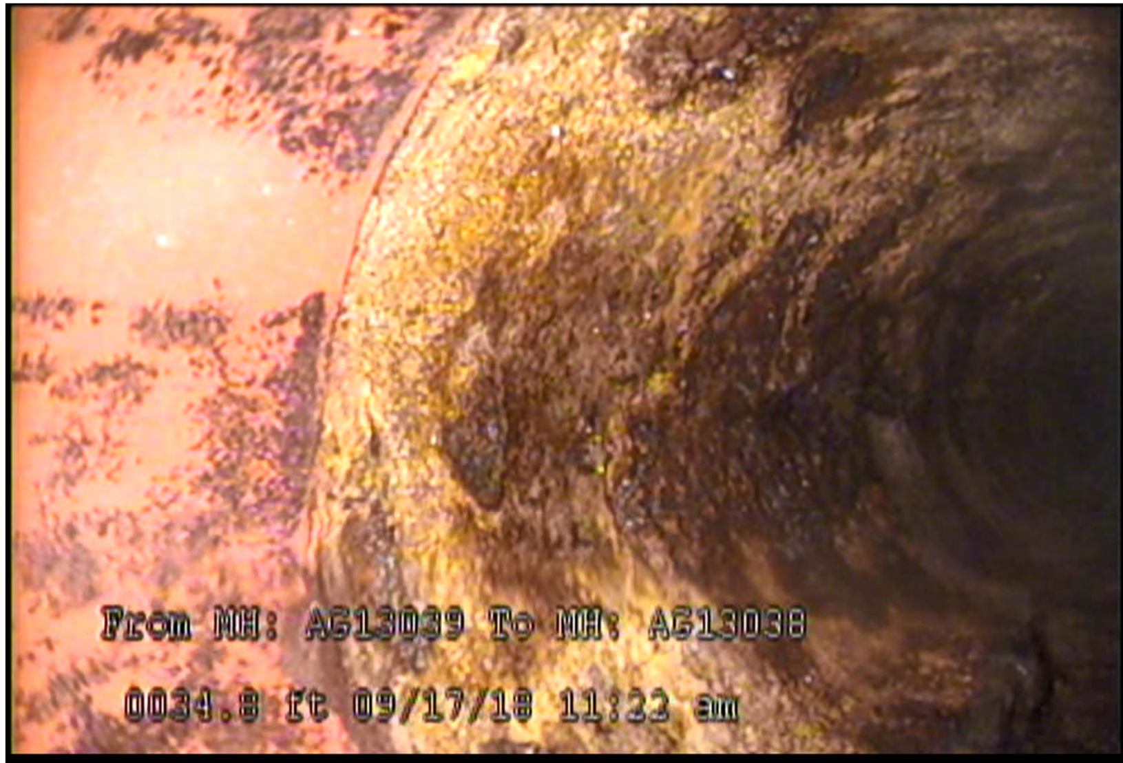
Figure 4 - Site No. 9, Perry Road, Union City; Observed corrosion.
