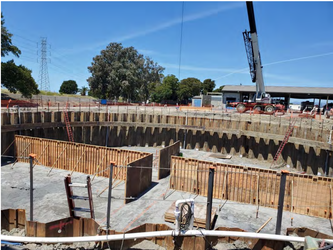
Image: Formwork Installation for Foundation Grade Beams
