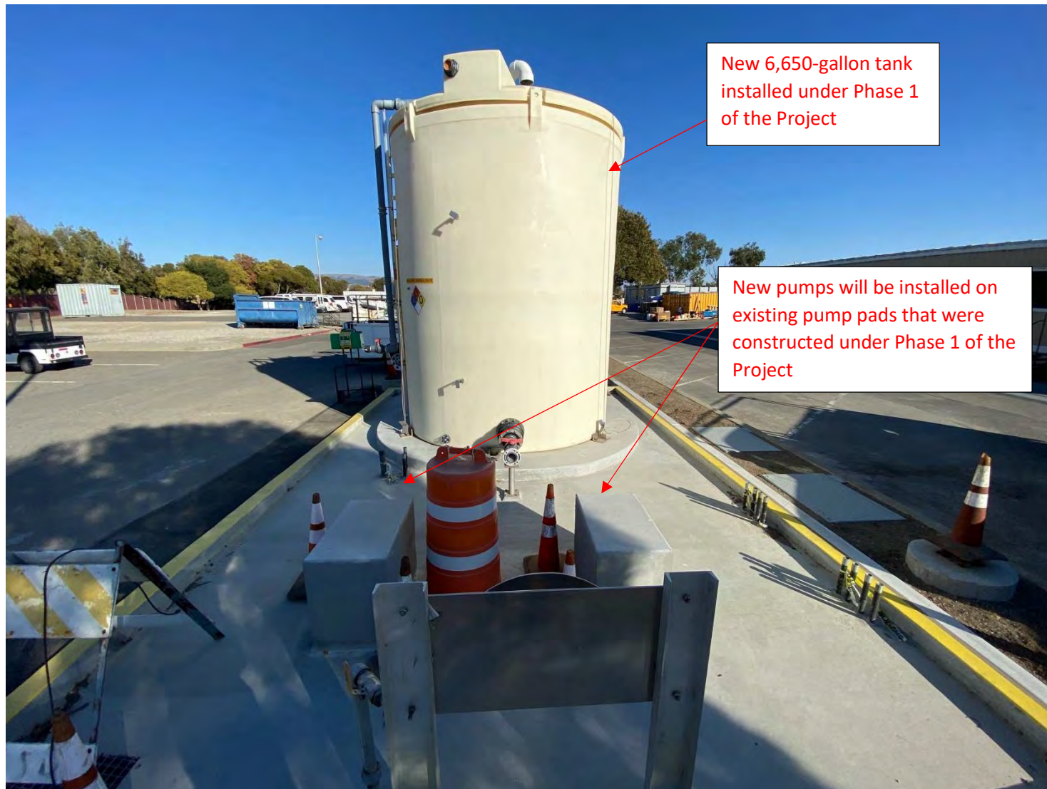
FIGURE 2 – Location of New Calcium Thiosulfate Pumps
