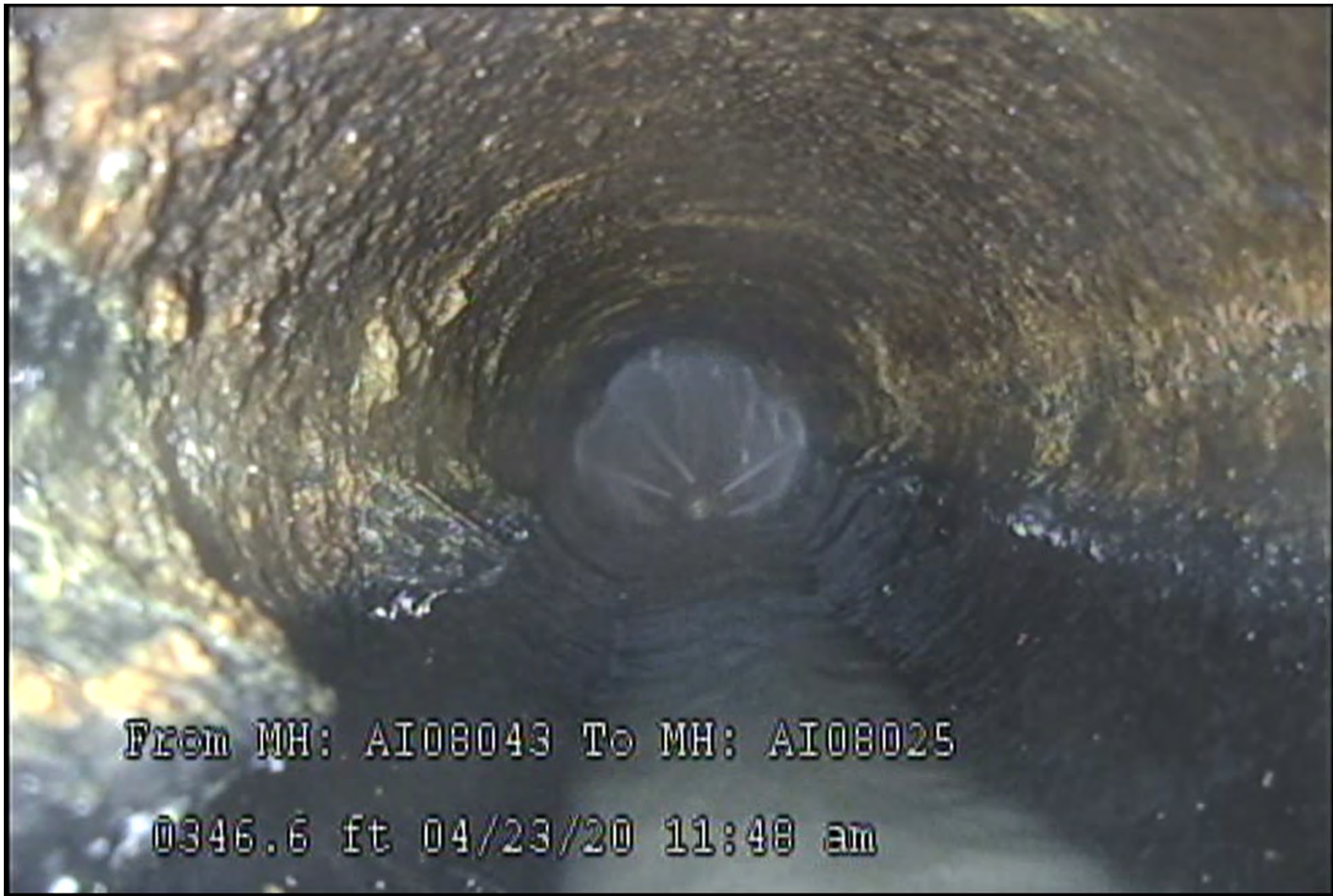
Figure 2 - Site No. 4B, Brier Street, Union City; Observed corrosion.
