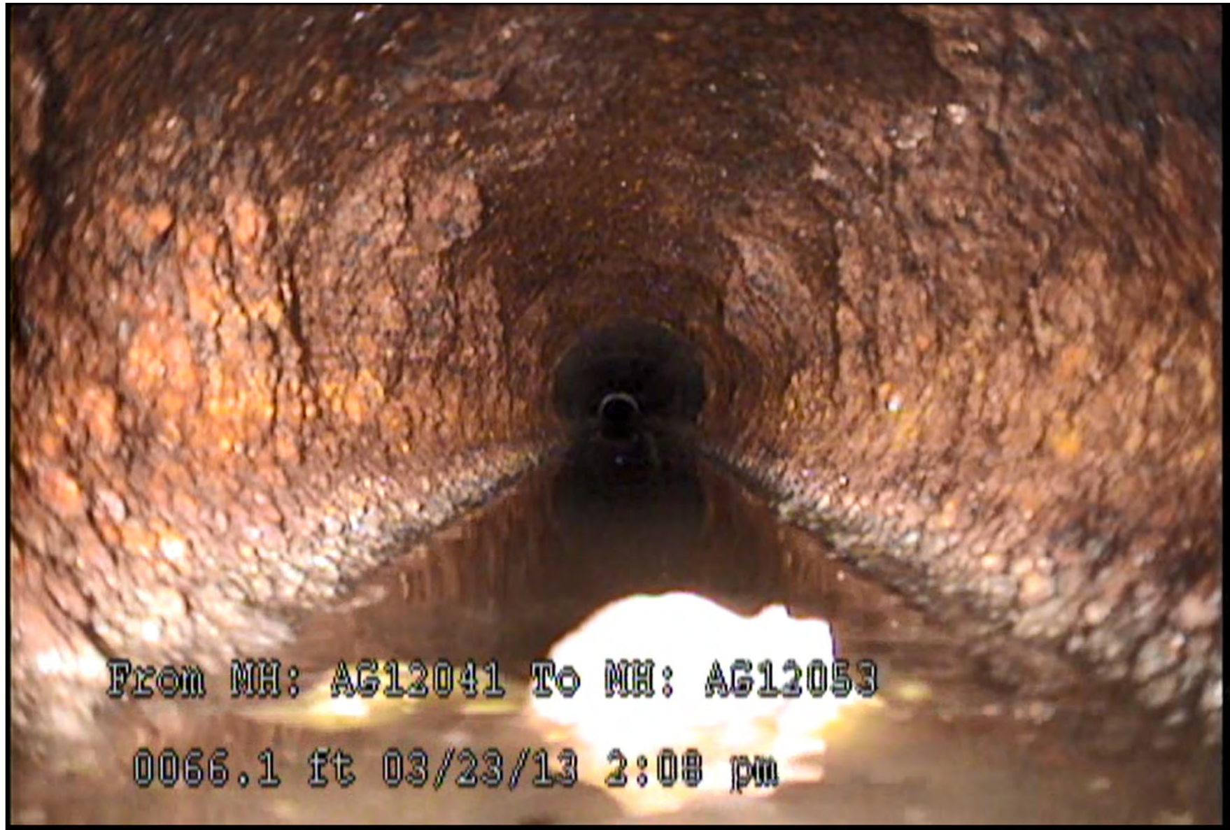
Figure 5 - Site No. 14, Alpine Court, Fremont; Observed corrosion.
