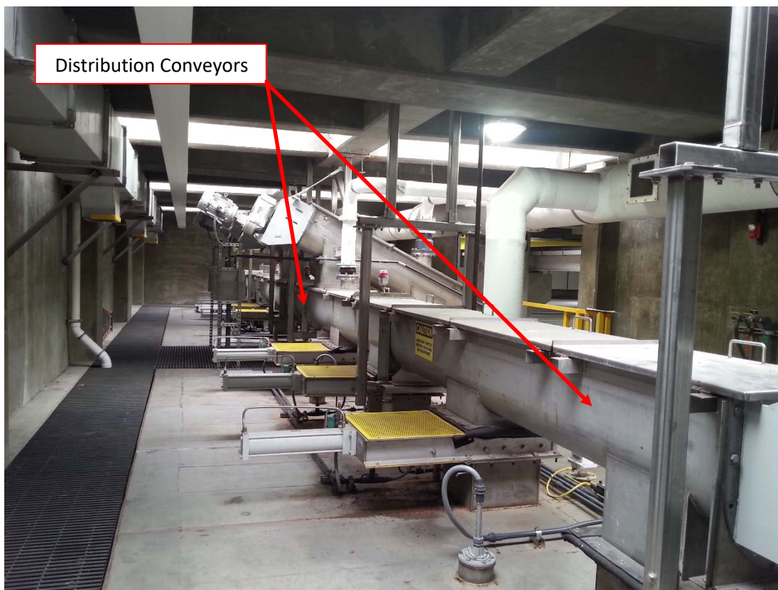
Figure 7 - Distribution Conveyors Over the Sludge Storage Hoppers
