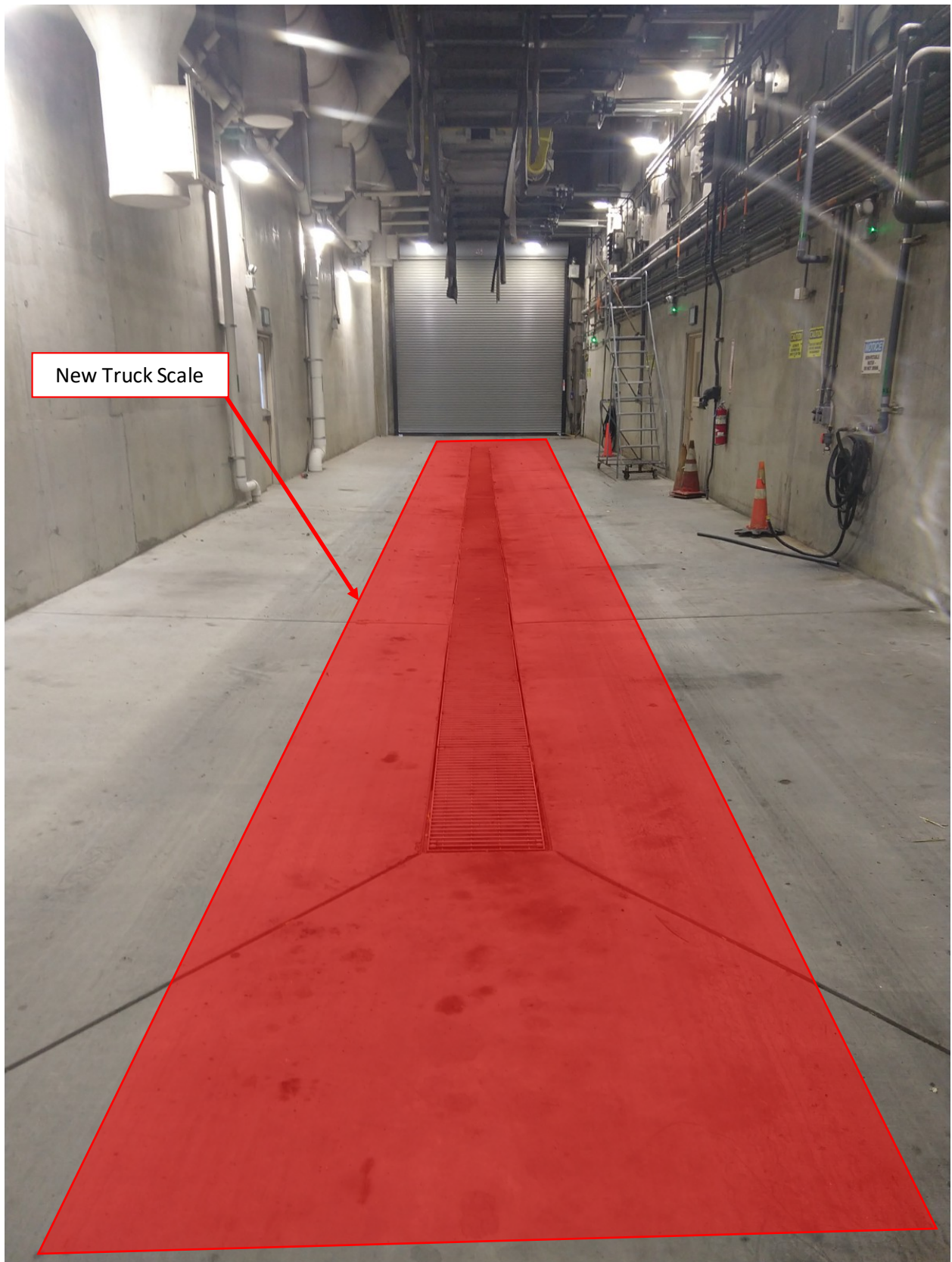
Figure 10 – New Truck Scale Inside Sludge Loadout Room
