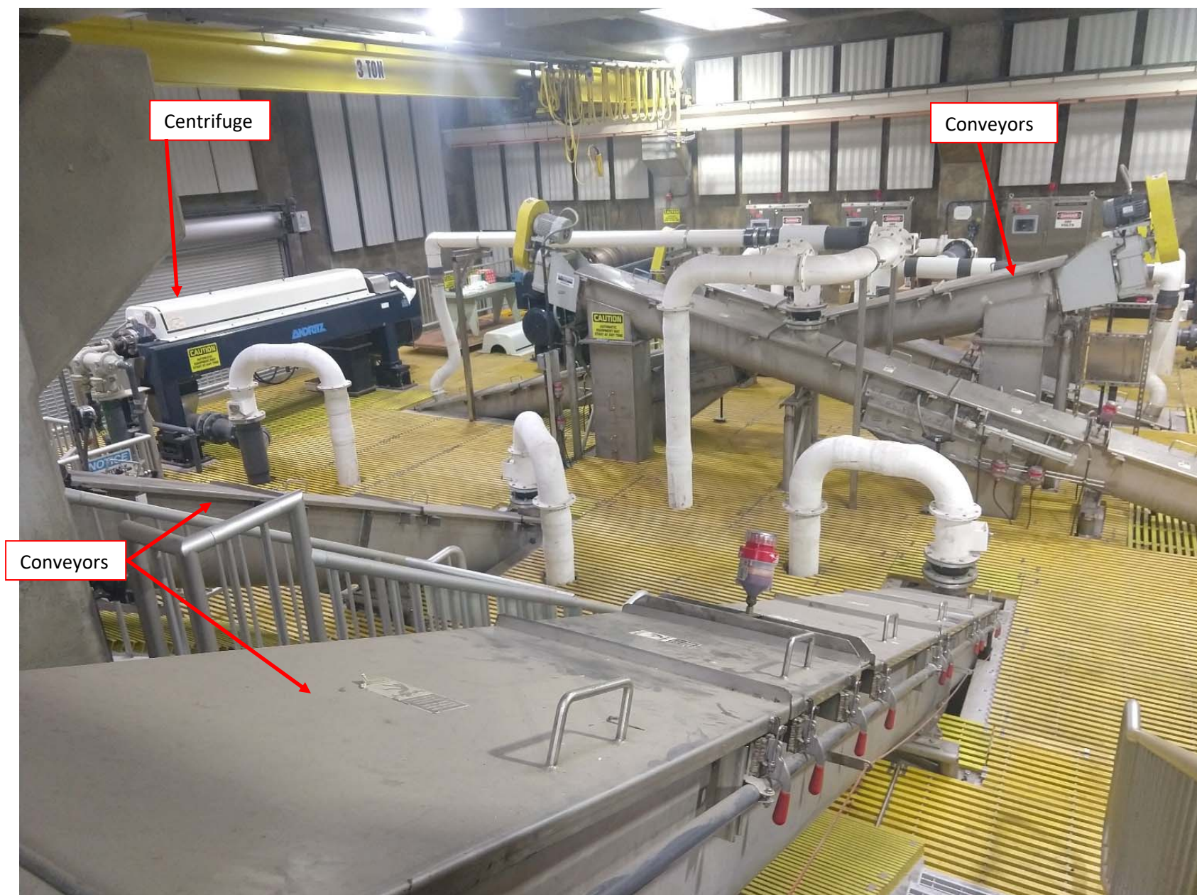
Figure 2 – Centrifuge Sludge Conveyance System
