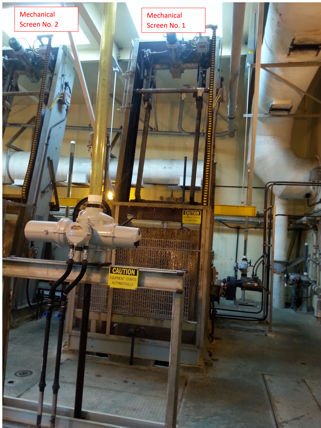
Figure 3 – Existing Headworks Screens No.1 and 2
