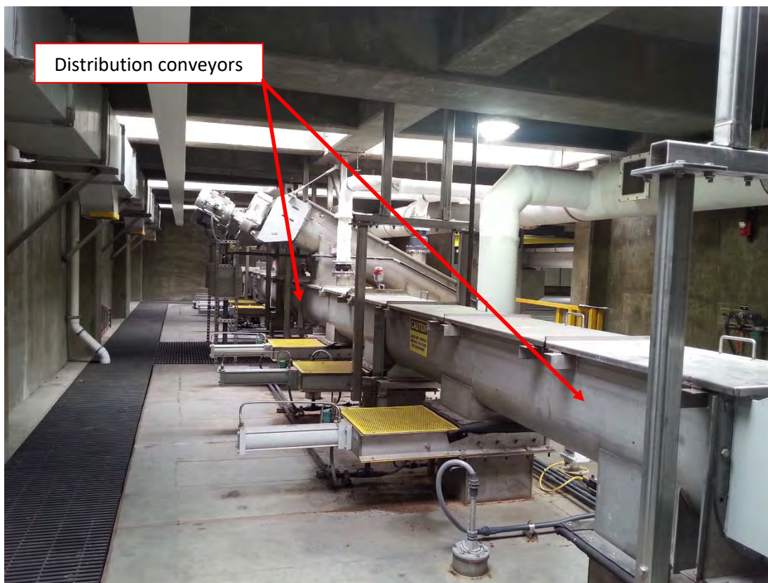
Figure 3 - Distribution conveyors over the Sludge Storage Hoppers
