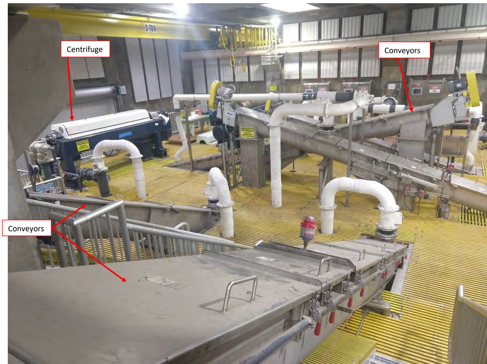
Figure 2 – Centrifuge Sludge Conveyance System
