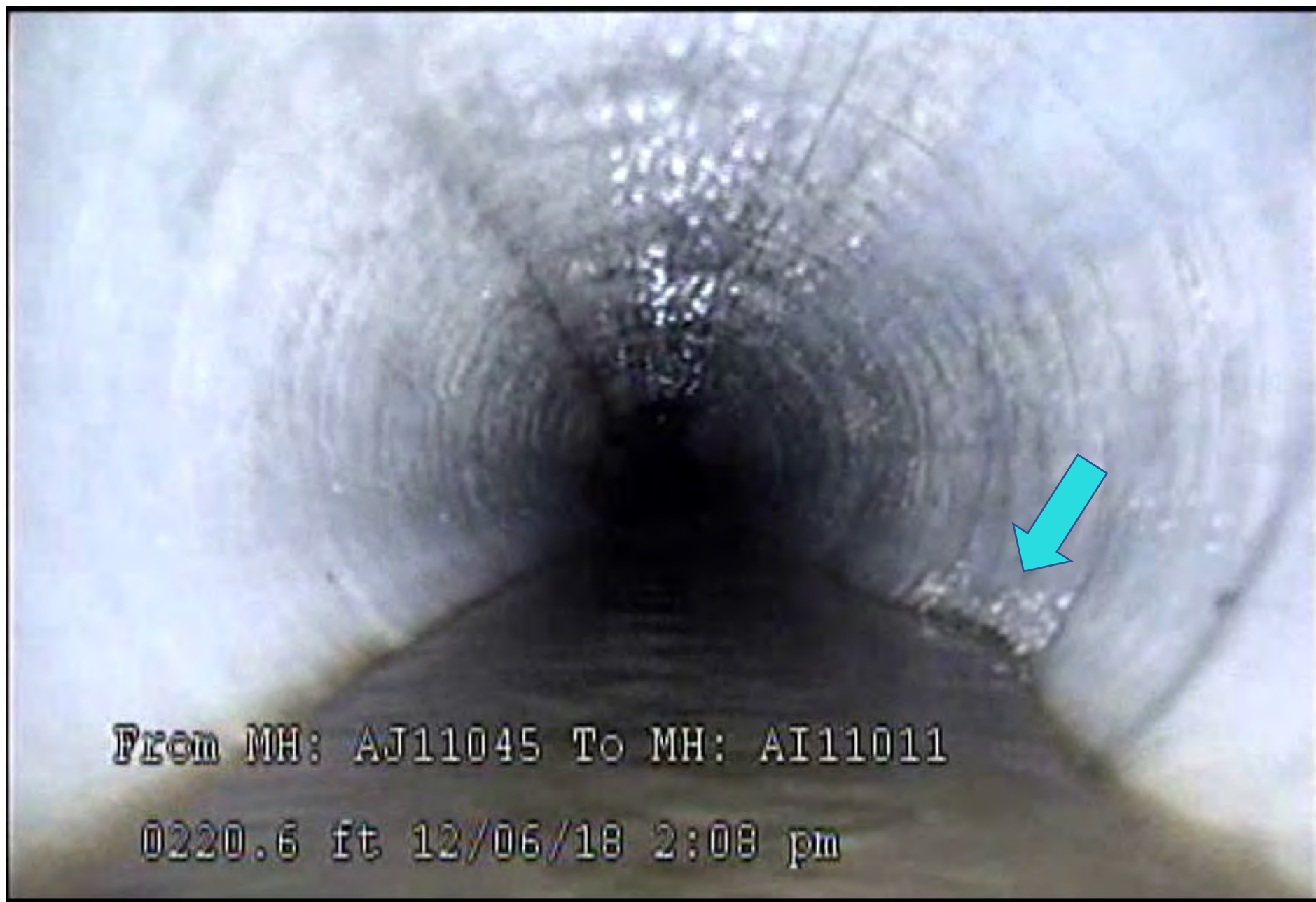
Figure 3 – Site No. 9, Hop Ranch Road, Union City; After CIPP Liner Installation
