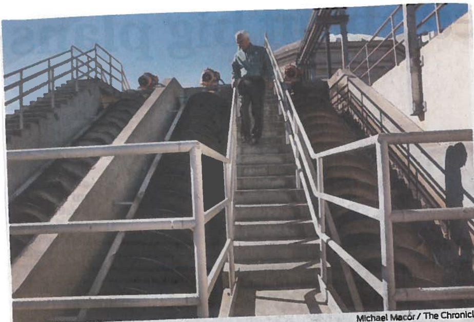
General Manager Gary Darling walks past giant augers that transport dirty water to aeration tanks above at Delta Diablo's recycling plant in Antioch.
